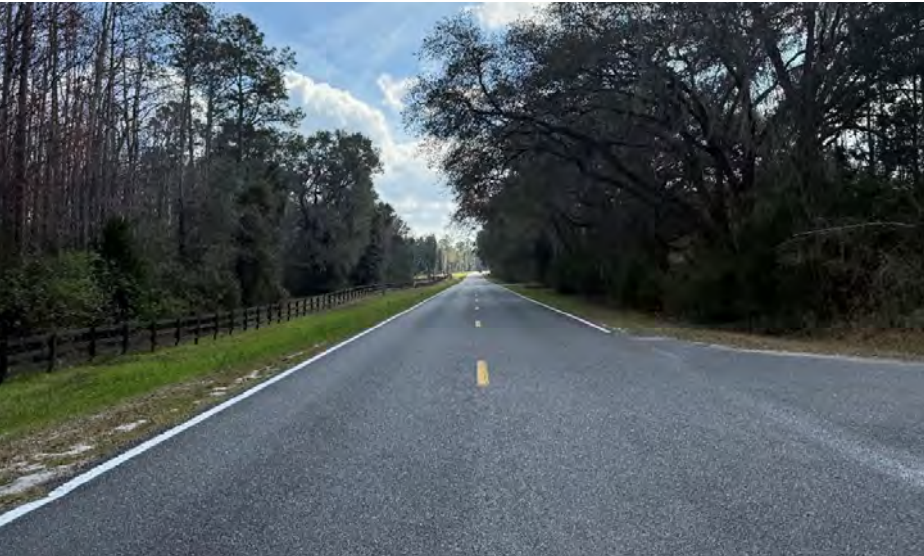
SW TUSTENUGGEE AVENUE (FACING SOUTH)
