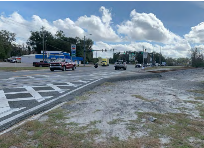
PAVEMENT EXTENDING BEYOND ROADWAY WITH TRAIN TRACKS
