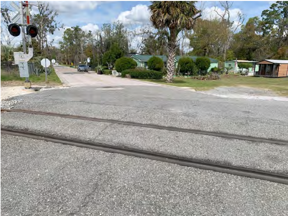
SOUTHBOUND STOP BAR AT RAILROAD CROSSING
