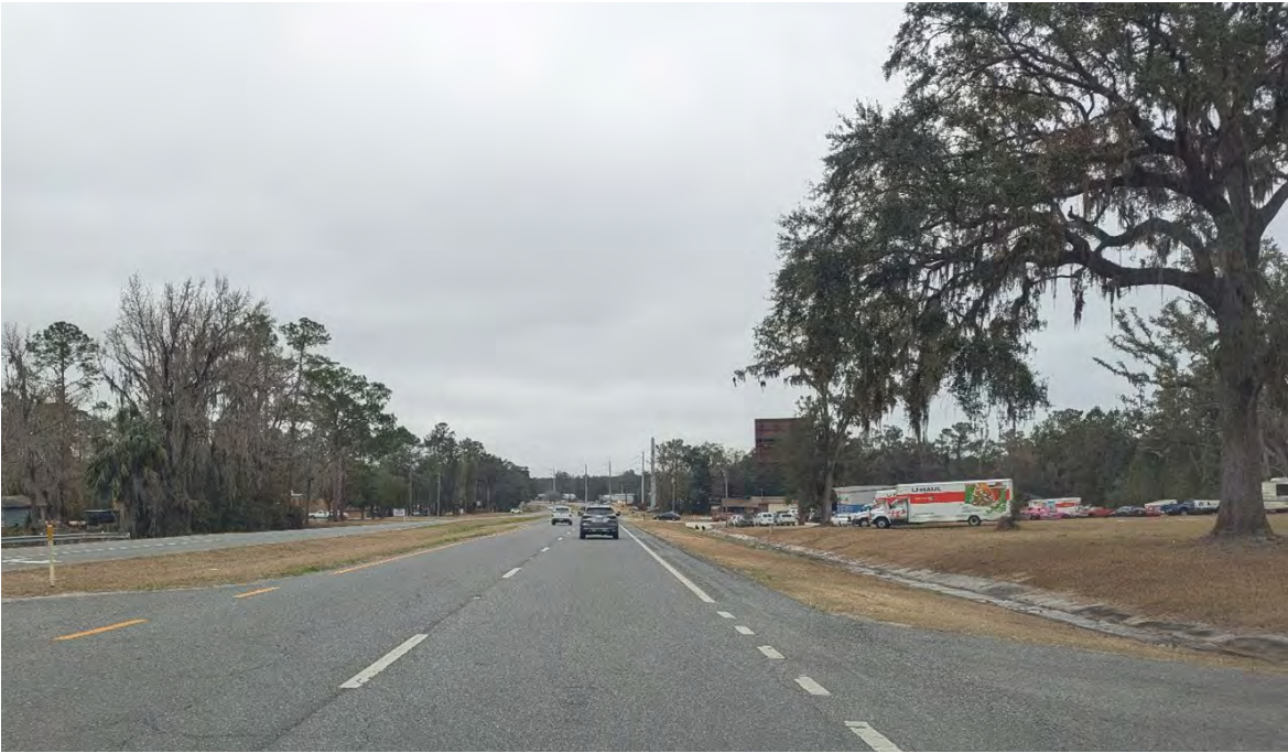
LACK OF LIGHTING
