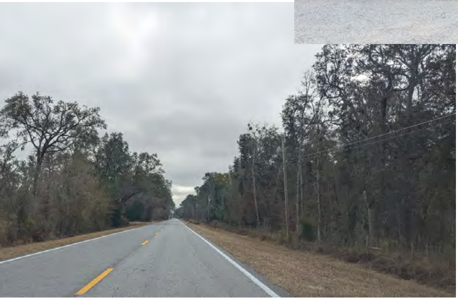
UTILITY LINES FOR POTENTIAL LIGHTING IMPROVEMENTS
