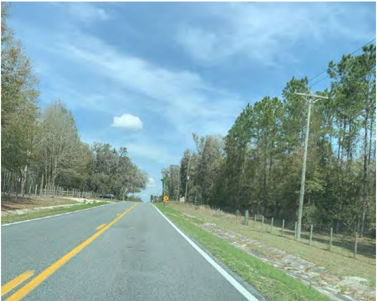
LACK OF LIGHTING ALONG SW TUSTENUGGEE AVENUE
