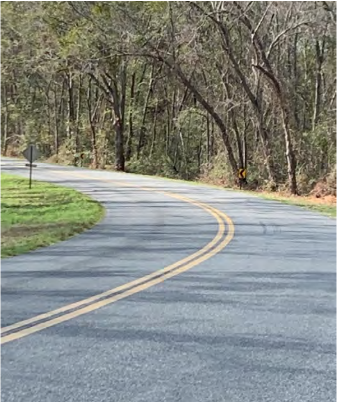
CHEVRON SIGNS ON NORTHERN CURVE
