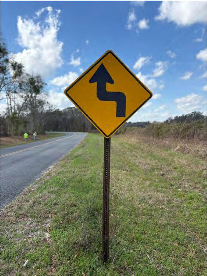
ADVANCE WARNING OF CURVE SIGN
