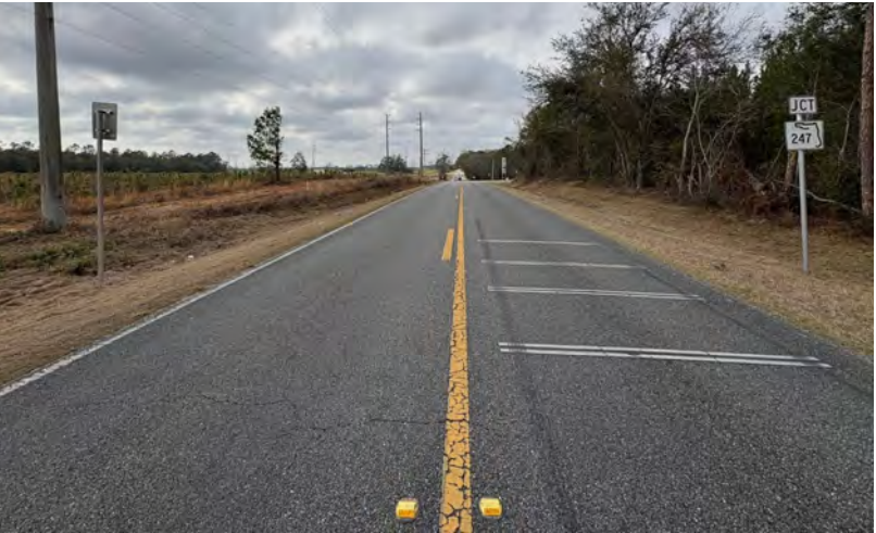
WESTBOUND APPROACH TRANSVERSE RUMBLE STRIPS
