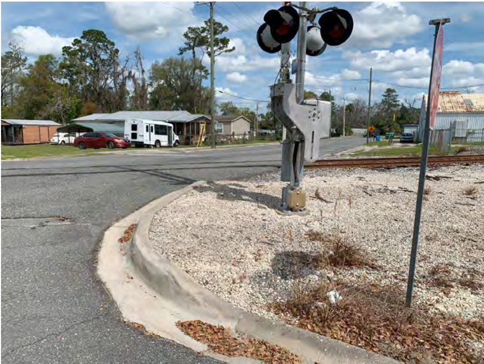
RAILROAD CROSSING ON NW LONG STREET
