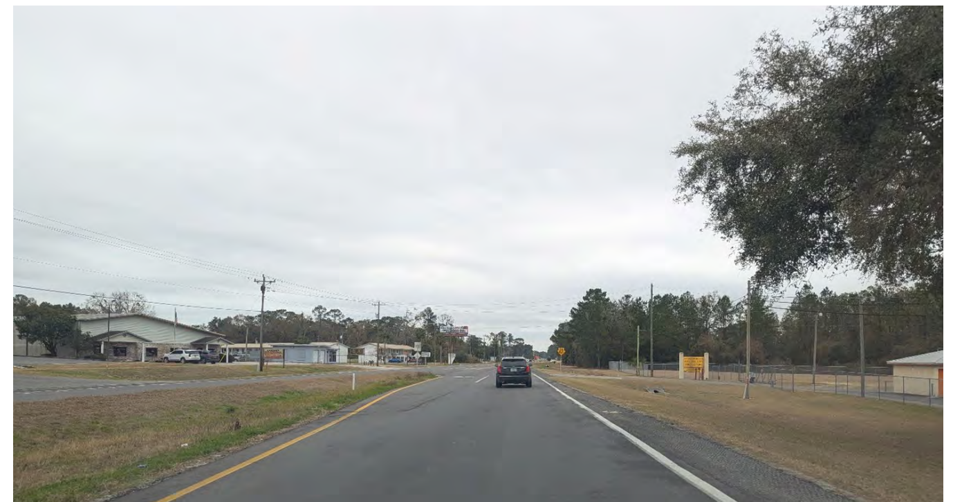
LACK OF LIGHTING
