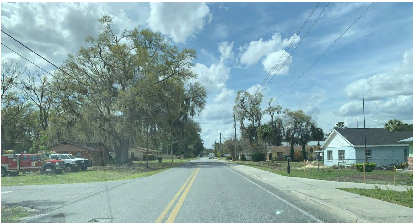
CURB IS INCONSISTENT ALONG ROADWAY
