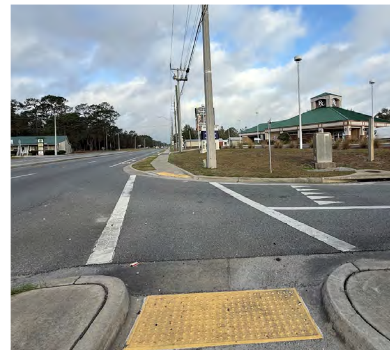
MISSING PEDESTRIAN MARKINGS ON NORTHERN LEG
