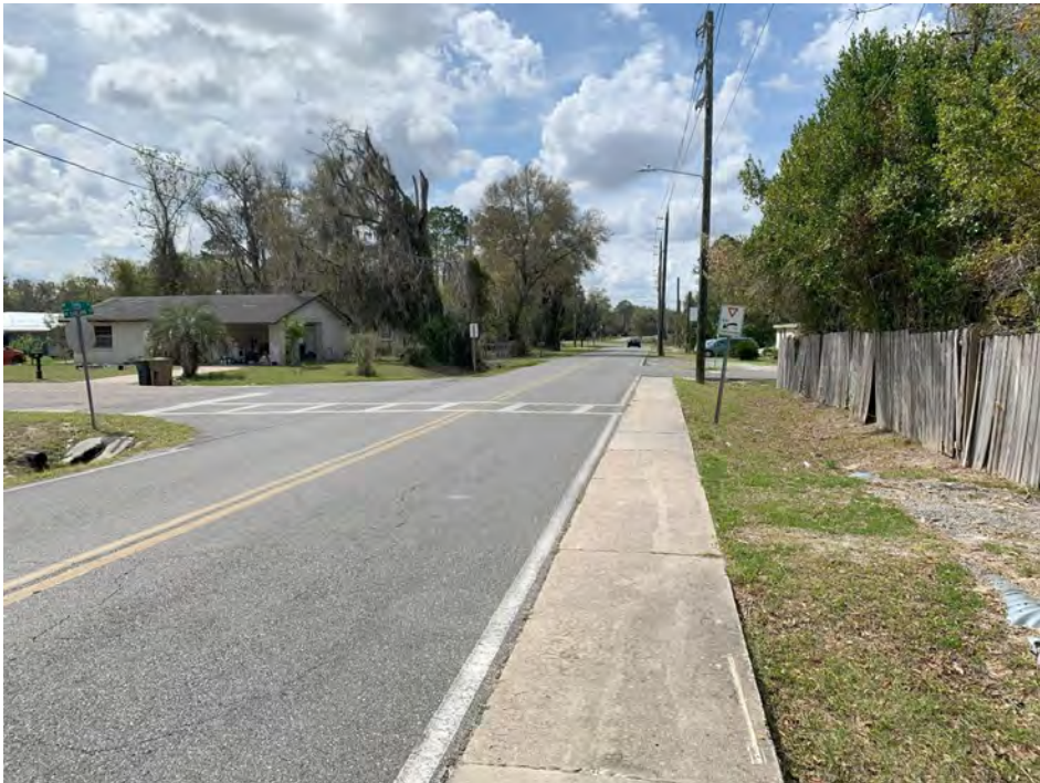
CROSSWALK HAS MINIMAL SIGNAGE
