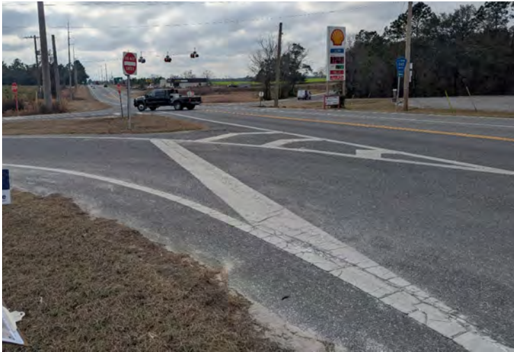
SOUTHBOUND LEFT IS A TIGHT ANGLE
