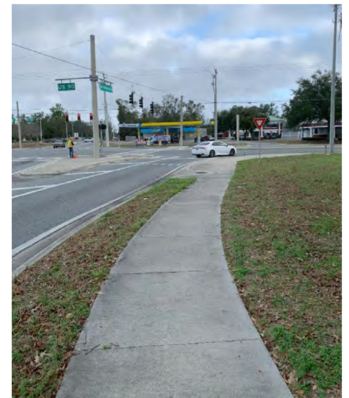
VIEW OF CHANNELIZED RIGHT TURN ISLAND
