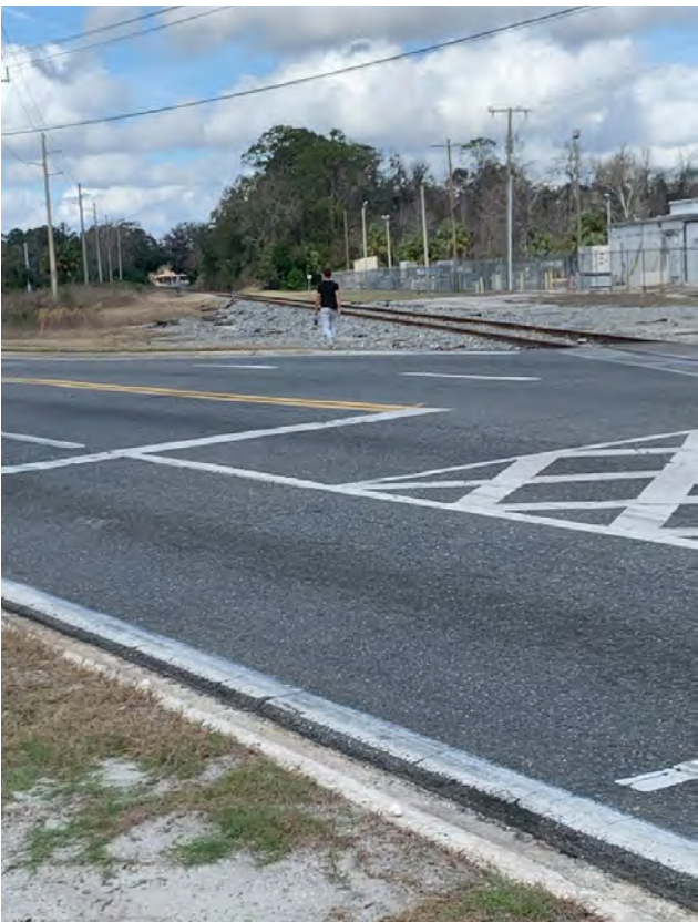
PEDESTRIAN NEAR TRAIN TRACKS WITHOUT PROPER FACILITIES
