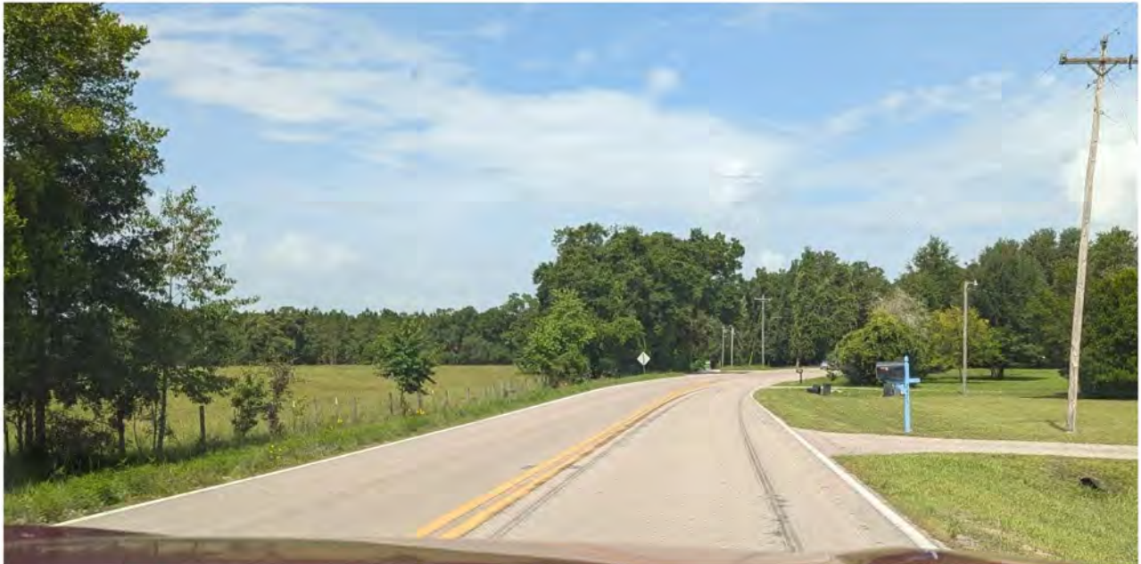
Westbound approaching Southern "Curve 2"
