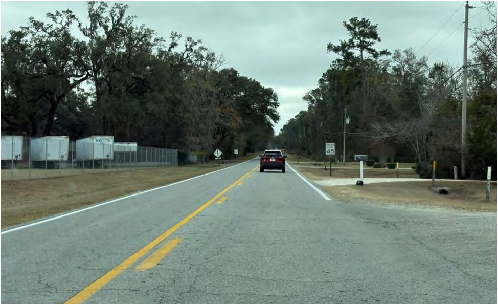
SW TUSTENUGGEE AVENUE (FACING SOUTH)
